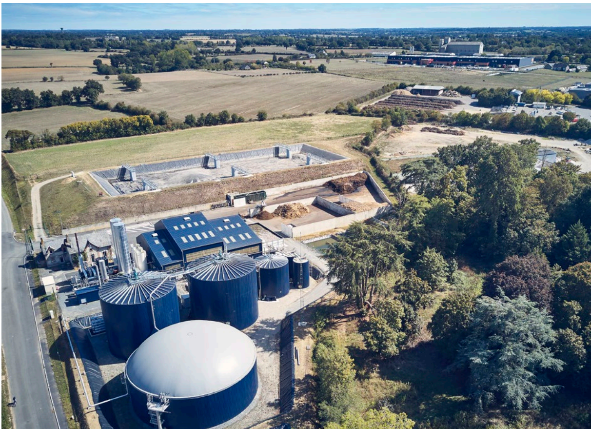
Evergaz biomass plant, Château Gontier, France
