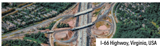
I-66 Highway, Virginia, USA
