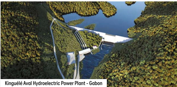
Kinguélé Aval Hydroelectric Power Plant - Gabon
